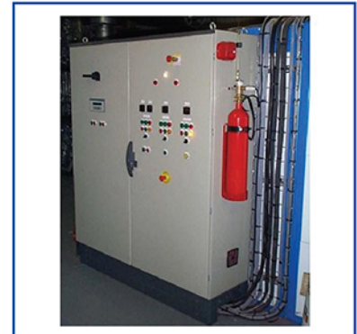
Electrical-cabinet-fire-protection
